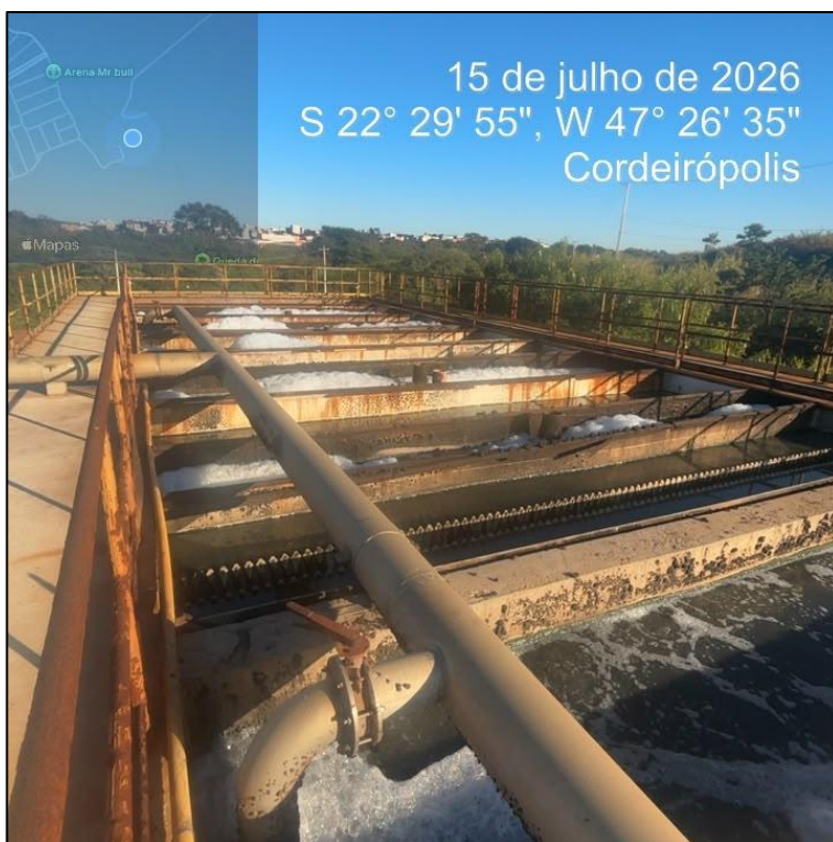
(b) Reator UASB.
